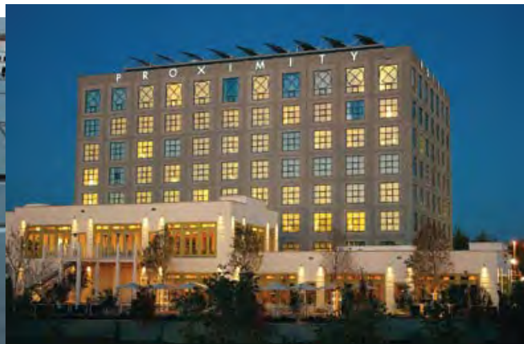
The Proximity Hotel, located in Greensboro, N.C., is currently in LEED's review process, but believes it will be the first certified Platinum hotel in the country.
